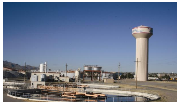
Figure 6. Haskell Street Wastewater Treatment Plant (Source: El Paso Water Utilities)
