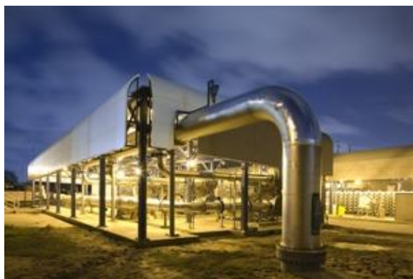
Figure 17. Edward C. Little Water Recycling Facility, El Segundo, CA (Source: West Basin Municipal Utility District)
